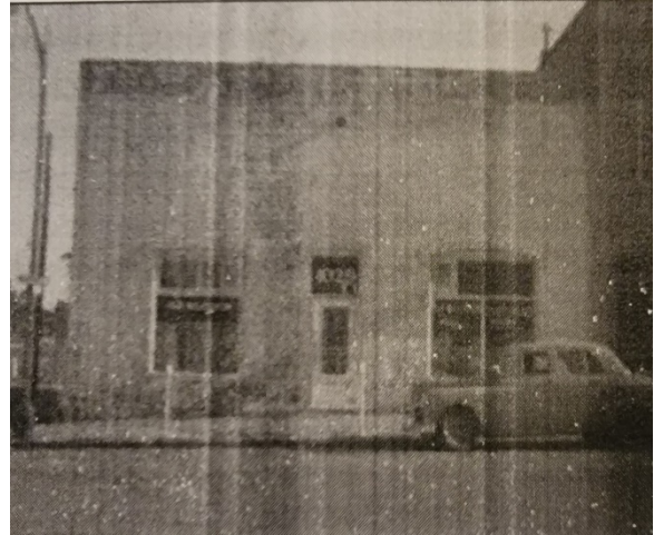
1840 Building at 11th and Franklin Lexington MO
